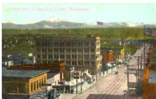
Hewitt Avenue looking east, Everett
