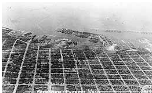
Aerial view of Everett, 1950s
