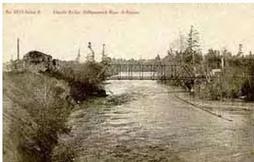
Lincoln Bridge, Stillaguamish River, Arlington, 1900s
